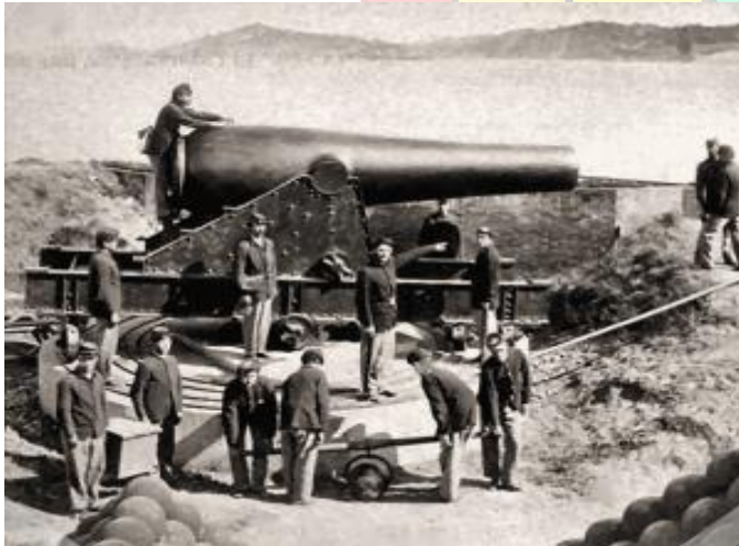
Alcatraz, 1870, a 15 inch Rodman muzzle-loaded smoothbore cannon that shot solid cannonballs.
